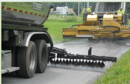
Binder and Chipseal application.
